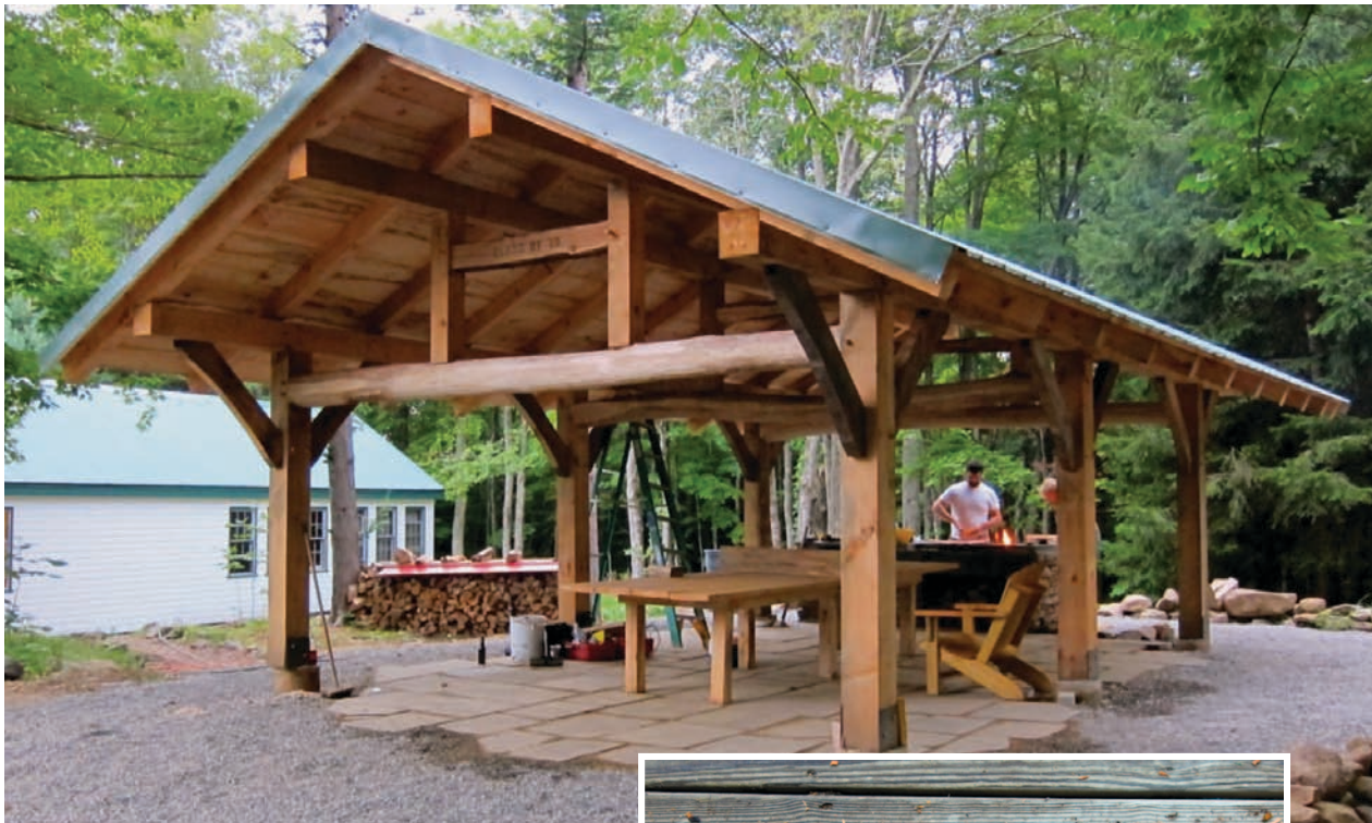
Yale-Myers Timber Pavilion, erected 2011
