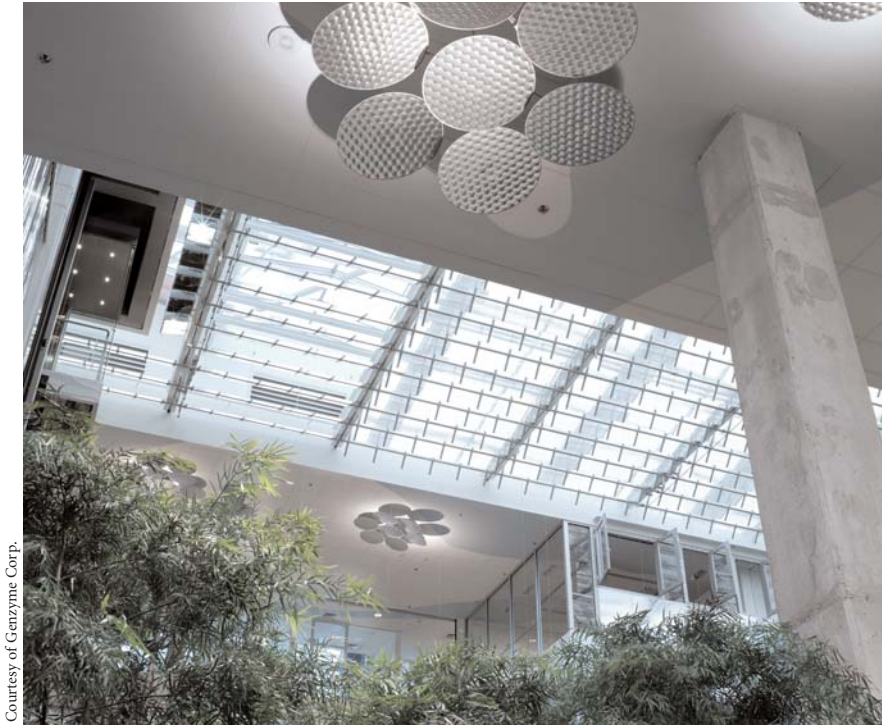
The louvered panels below the skylight and the florets above the interior garden diffuse harsh light and reflect and distribute soft light into the interior of the Genzyme Center in Cambridge, Mass.
